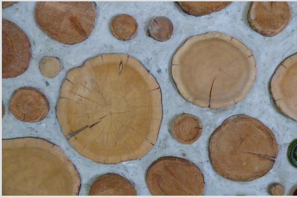
A closeup of cordwood masonry, a natural building method used on The Farm.
