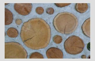
A closeup of cordword masonry, a natural building method used on The Farm.
